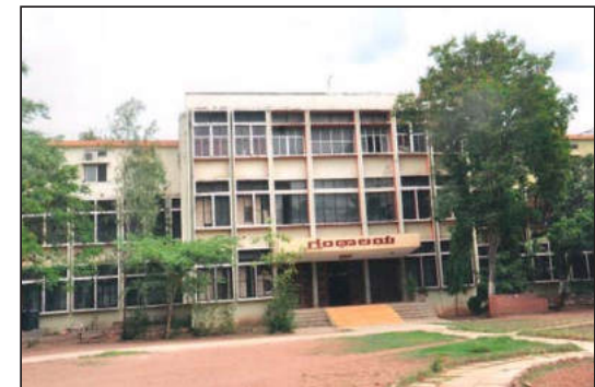
Front view of Library
